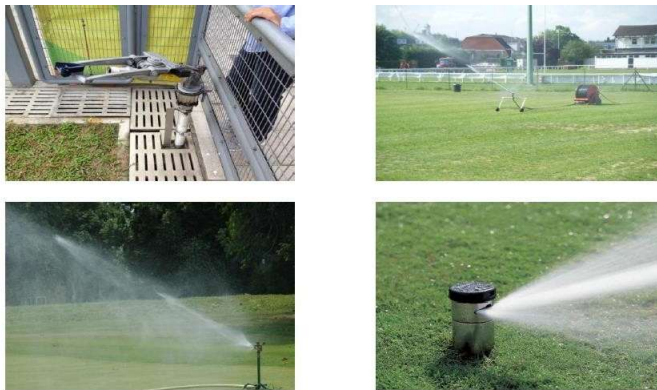
Fig. 3. Types of irrigation systems used in the sports turf industry. From left to right: canon type, self-travelling type, static type and pop-up type. Only automatic pop-up irrigation systems are considered appropriate for pitches
